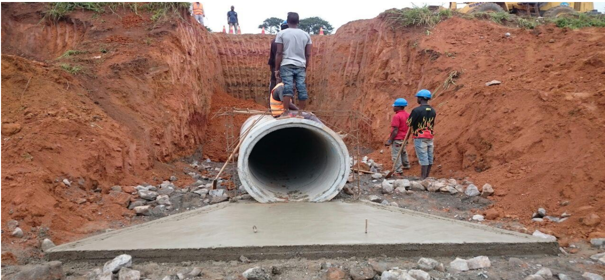
Culvert installation along the road
