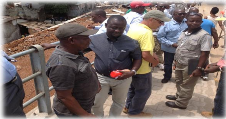
The Newly reconstructed King Jimmy Bridge
