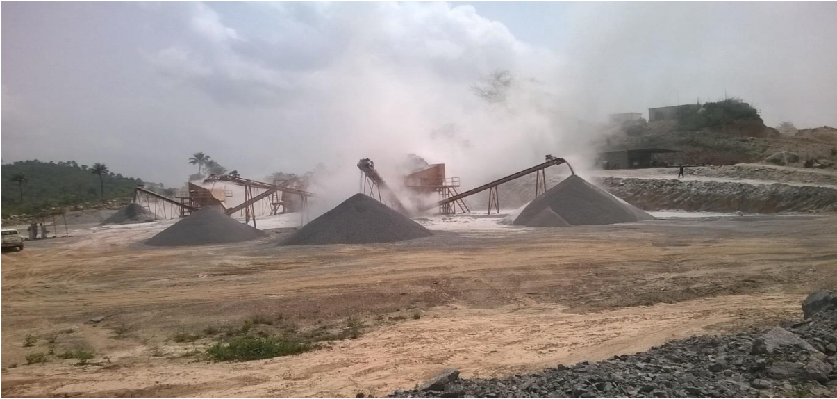
Crusher plant completely installed and in full operation
