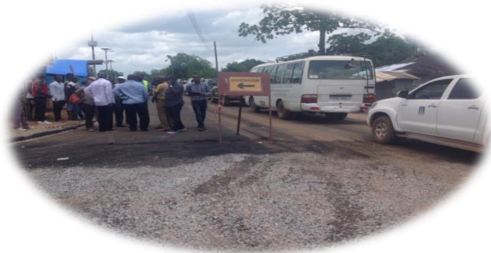
Pujehun Township roadworks
