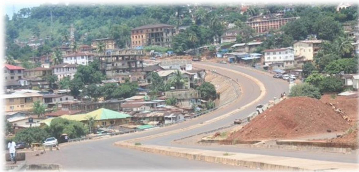
Completed roadworks on the Hill Side By-pass road
