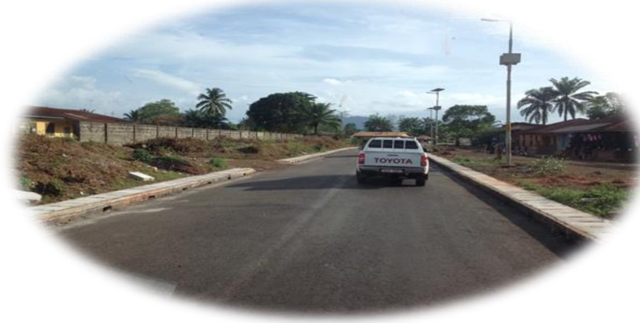
Completed roadworks on Moyamba Township
